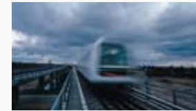
Driverless Metro System
